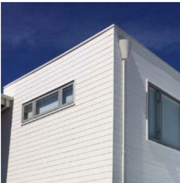
2 WEATHERTEX : ECOGROOVE SMOOTH 300MM COLOR: DULUX FLAT WHITE
